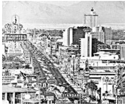
figure 36. Upper Strip looking North
